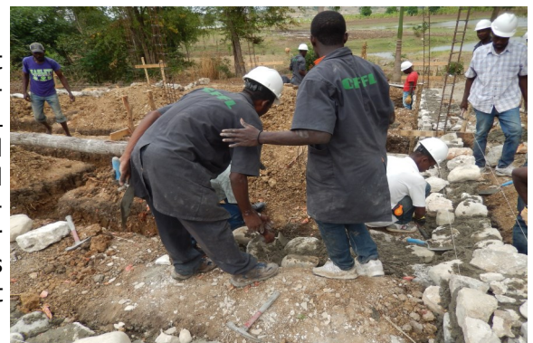
Students Work on VFHI Building Foundation.
